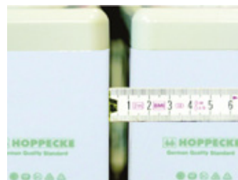
Fig. 5-14: 10 mm clearance between the batteries
