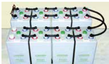
Fig. 5-15: Using row connectors and step connectors
